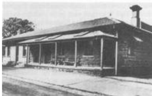
FIGURE 2. The original Victoria Barracks Laboratory Building
